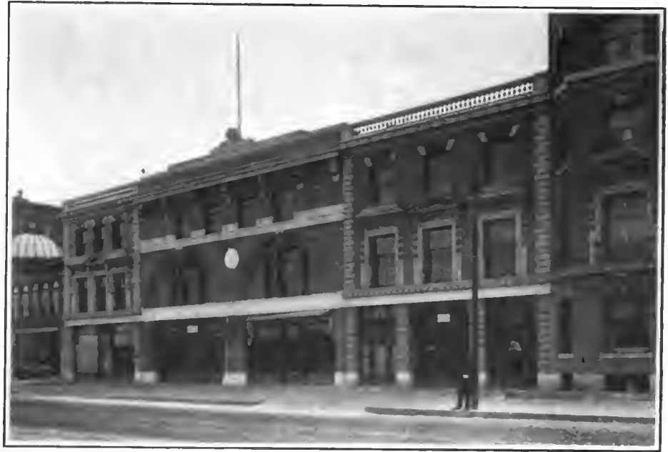
MASSACHUSETTS A. C. CLUBHOUSE, BOYLSTON STREET, BOSTON. SHOWING NEW EXTENSION.
